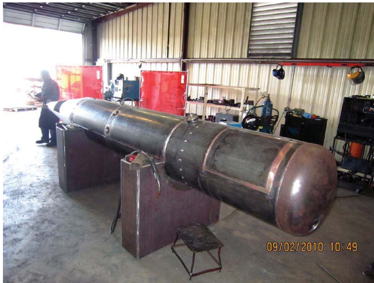
50 Holes drilled for the Stainless Steel Rivets
